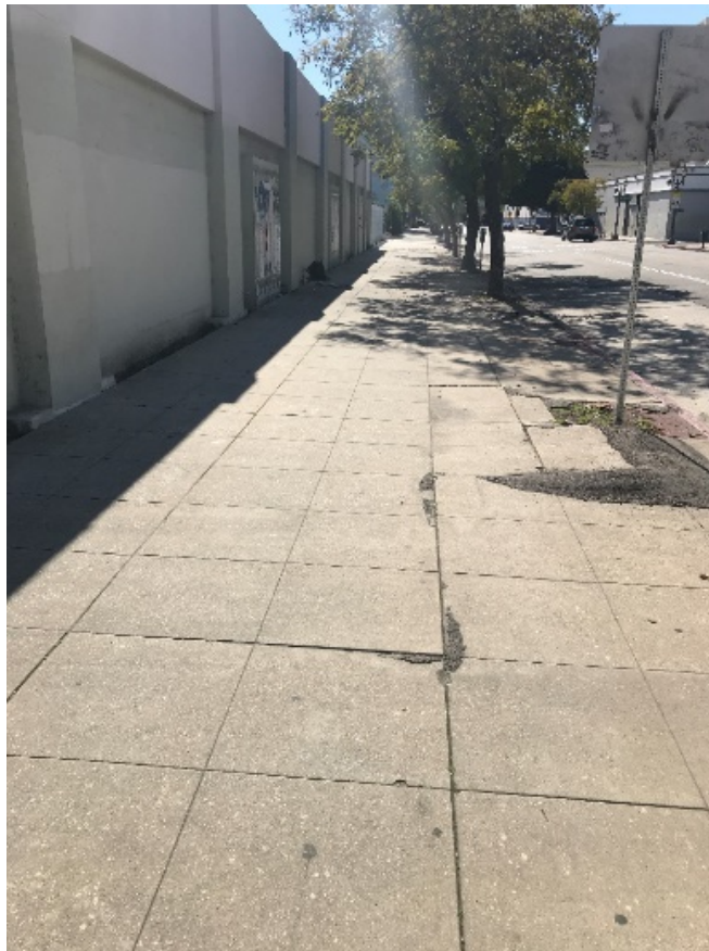
Figure 6: Wide sidewalk with unevenness that leaves >4 ft. of passable width (block group 3, Fashion District)
